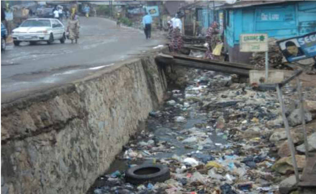
Plate 4.5: An Overview of Dumped Solid Waste in the Open Drains in Oje Market
